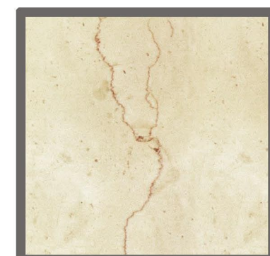
Interior details: Marble panels-Beige
