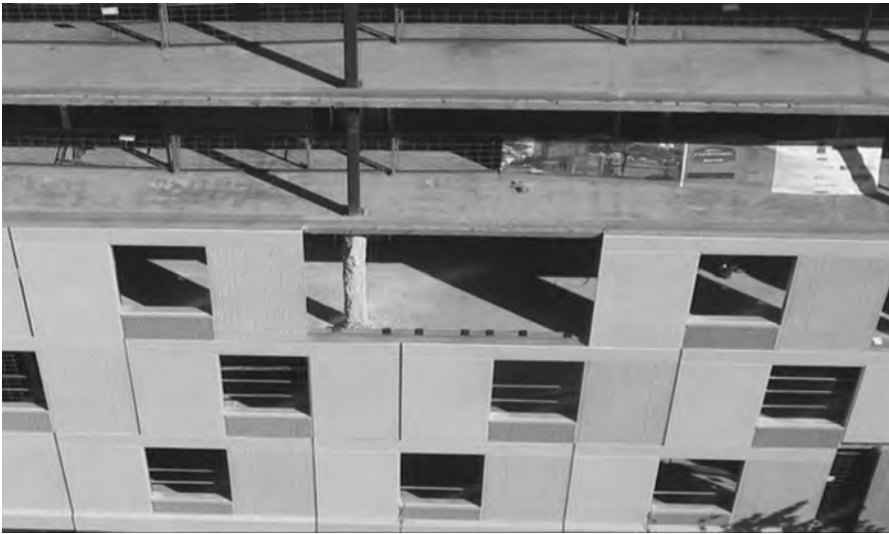
FIGURE 9-2-9 Precast panel installation process.
