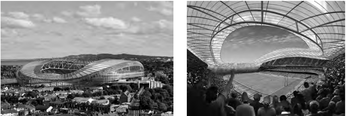
FIGURE 9-1-2 (Left) A view of the finished stadium. (Right) A view of approved configuration from stadium seats with Dublin skyline in background. (See color insert for full color figure.)
